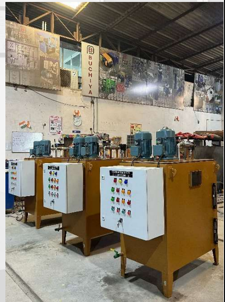
OIL LEAKAGE SYSTEMS
